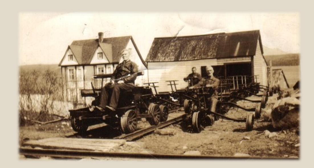
In 1920 the first hand pumps and velocipedes (a three-wheeled hand propelled track vehicle) were introduced. This continued as standard equipment until the early 1930's when the first powered pumps and powered rail cars (speeders) became part of the arsenal of equipment. The government authorized the establishment of the first fire lookout towers and construction was started in 1935. One of the first four towers was located at Mount Blandford, just to the southeast of Port Blandford.
